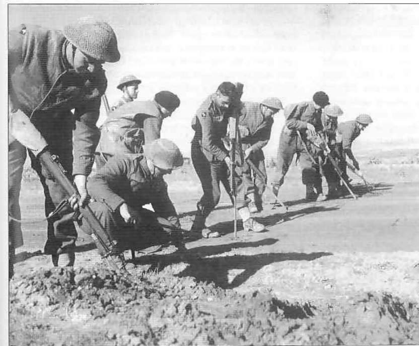
As the desert war went on and mines proliferated, the clearance of minefields grew inexorably in importance – see Plate F. Here men of 6th Arm'd Div are using the basic search method – prodding with bayonets – on the Thala-Kasserine road, Tunisia, on 24 February 1943. Prodding was a slow, nerve-wracking and manpower-intensive method; but although by Second Alamein electronic mine-detectors had arrived and a systematic doctrine had evolved for gapping even the largest minefields, an alert eye and a practised hand for prodding remained an essential first part of the process – as it does even today. (IWM NA 856)
